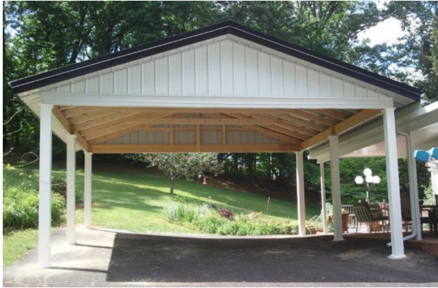
Acceptable – Service Line is Ventilated
