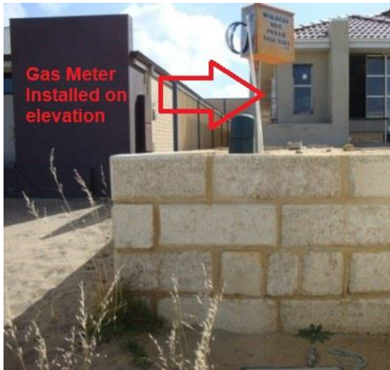
Not Acceptable – Location A
