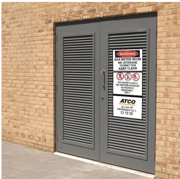
Figure 57: Meter Room – Example of Signage
