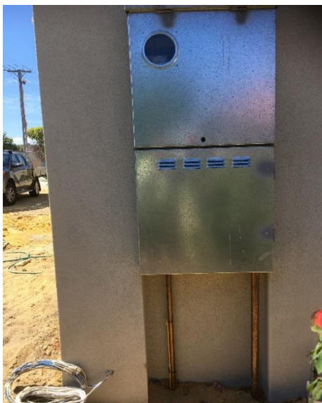
Conforming Installation (Recess Sealed from Cavity)
